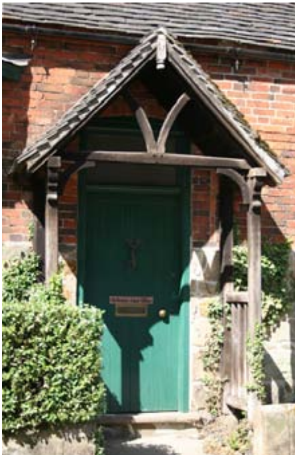
Left - the estate office to Melbourne Hall was adapted and up-dated in the early 20th century, along with a number of estate properties, using Arts & Crafts timber-frame details. The oak porch with arched braces is typical of this style.
