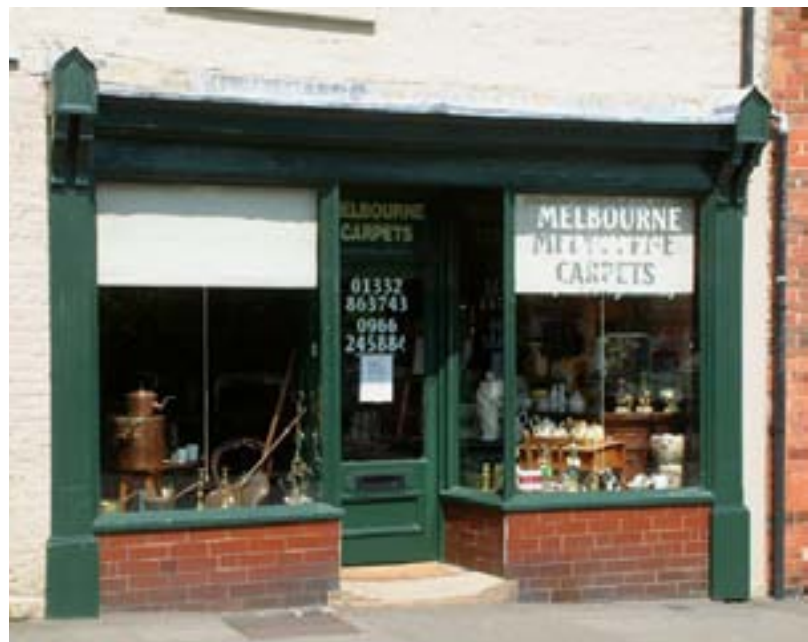
Right - Victorian shopfront at 38 High Street with brown glazed brick stall riser, decorative fluted pilasters with raised console brackets, recessed shop doorway, cornice and fascia.
