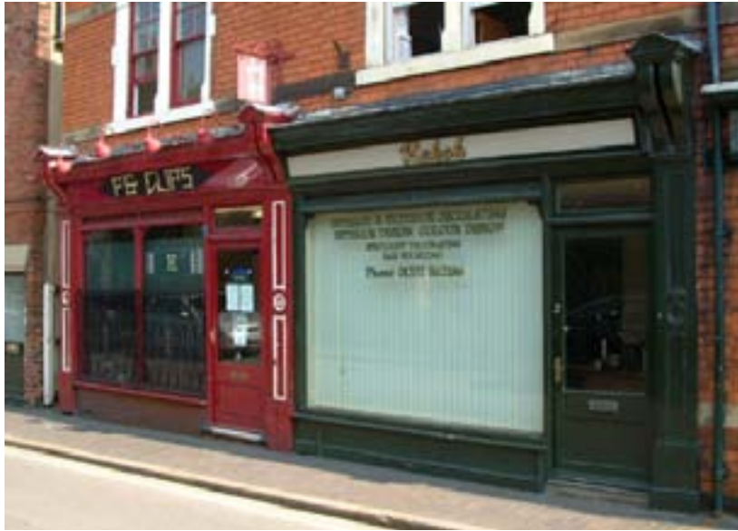
Left - late Victorian pair of identical shopfronts at 8-10 Derby Road. Heavily-moulded panelled pilasters, a bold cornice with console brackets and shop doors with fanlights. The shopfronts retain the original ventilation grilles and timber spandrels, but No. 8 has lost its central glazing mullion.
