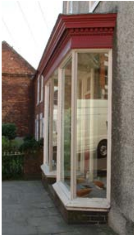
Left - refined projecting shopfront with intricate cornice, dentilled moulding & plate glass windows.
