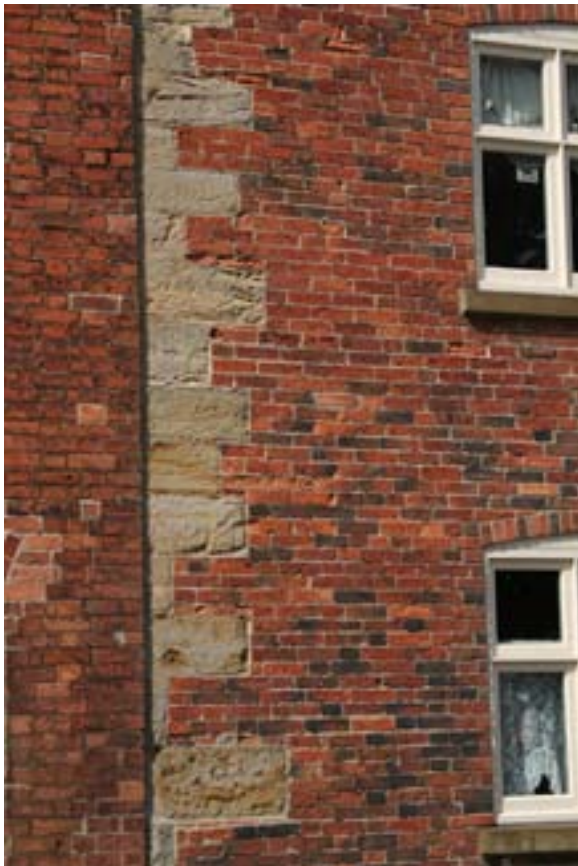
Below right - flush dressed stone quoins at Pool Cottage. The quoins were dressed in herringbone tooling with drafted margins. This is a highly decorative technique where the face of the stone was quartered and then each quarter separately tooled to create a herringbone pattern.
