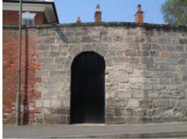
Above right - tall coursed gritstone walls at The Grange, Pack Horse Road (over 3 metres high)
