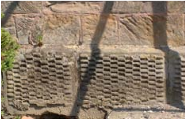
Above left - stone plinth with unusual chiselled tooling.
