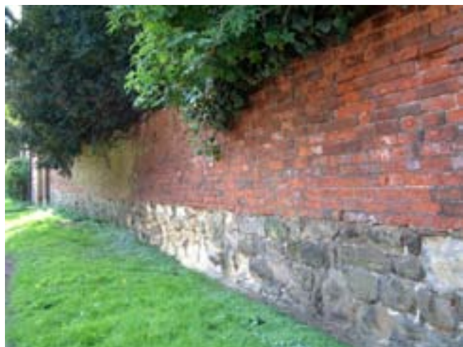
Below right - tall walls of red brick with an earlier stone wall used for footings at Chantry House, Church Street
