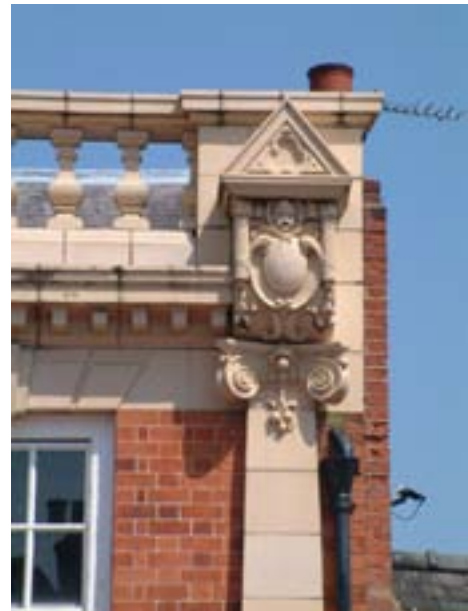
Below - bespoke buff architectural terracotta at the Co-op. The use of terracotta blossomed at the end of the 19th century.
