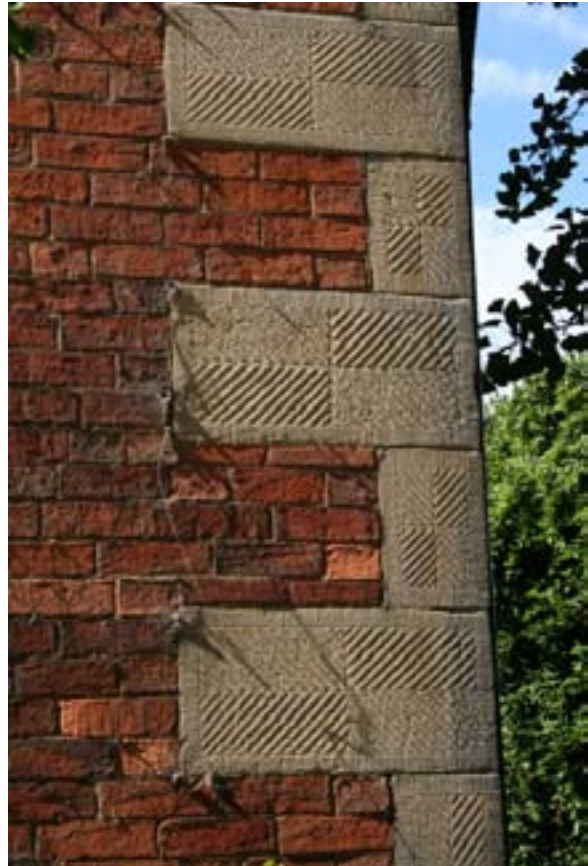
Below right - flush dressed stone quoins at Pool Cottage. The quoins were dressed in herringbone tooling with drafted margins. This is a highly decorative technique where the face of the stone was quartered and then each quarter separately tooled to create a herringbone pattern.
