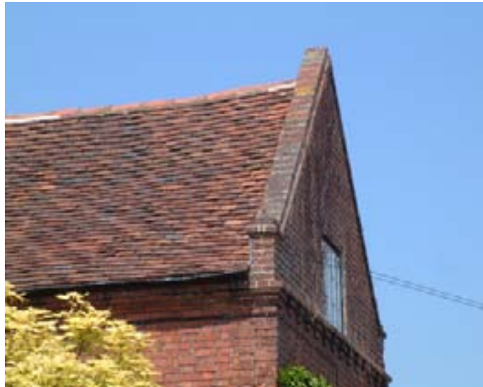
Above - raised coped brick gable. These were generally used on the higher status buildings during the mid-late 18th century.
