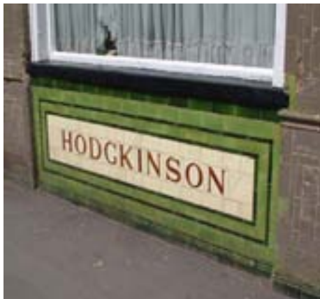
Below - tiled stall risers at 46 High Street & 7 Derby Road (bottom).
