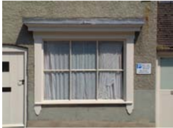
Right & above - 10 Market Place & 20 Potter Street - small "side street" shopfronts of the mid 19th century incorporating similar details; narrow pilasters, truncated at the base, a simple cornice and frieze rail and windows with glazing bars. The example at 20 Potter Street still retains its giant sash window.
