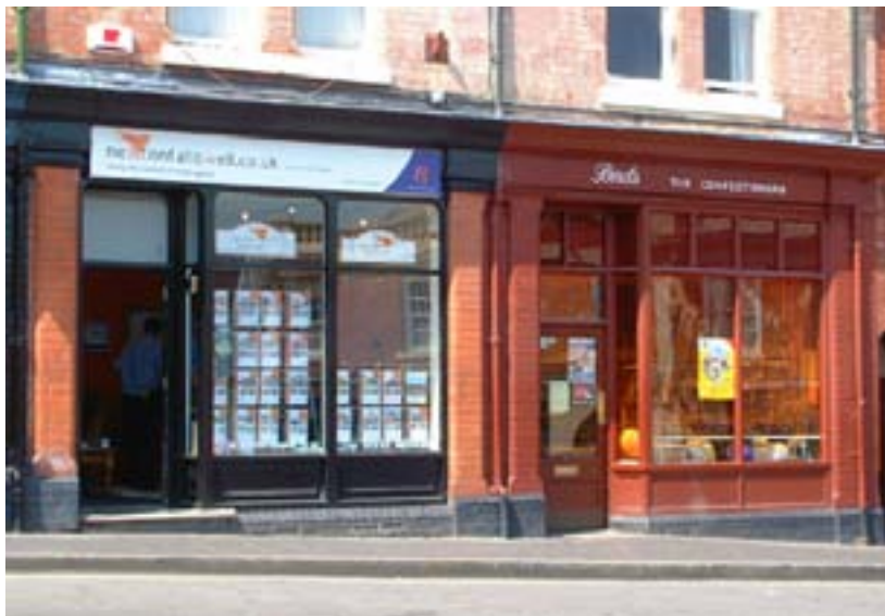
Left - Edwardian shopfronts at 31-32 Market Place, originally designed as two of three matching shopfronts. The pilasters were made from moulded red bricks (terracotta) and incorporate chamfers. The fascia and cornice was designed as one continuous run. The original style clerestory glazing survives at No. 32 (Birds).
