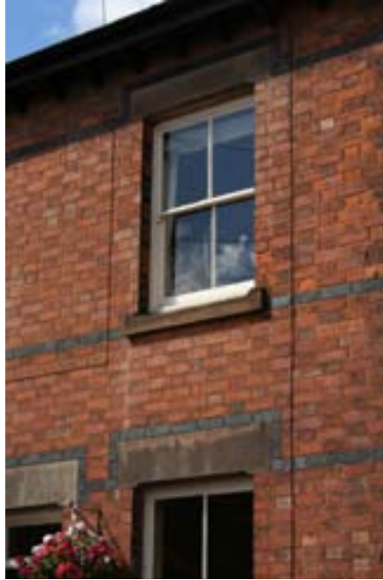
Left - polychromatic brickwork (the use of several colours of brick to create decorative patterns) used at 21 South Street (far left) & at 77 Castle Street (immediate left).
